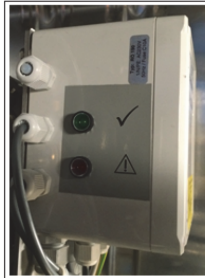
Fig. 12: LED signalling lamps on control device
