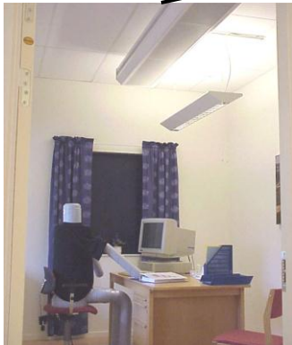
Office room - cooling coil - CAV - Air flow 15 l/s - Cooling capacity 700 W
