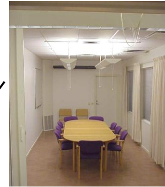
Conference room - VAV - Air flow 80 l/s - Cooling capacity 1200 W
