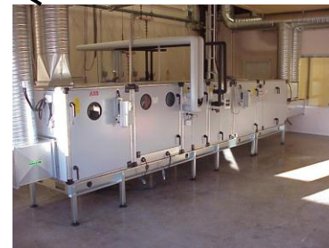
EC air handling unit with controls - Size 03 - Air flow 0,7 m 3 /s
